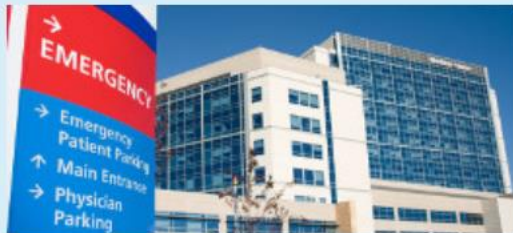
Acute Care Facility
